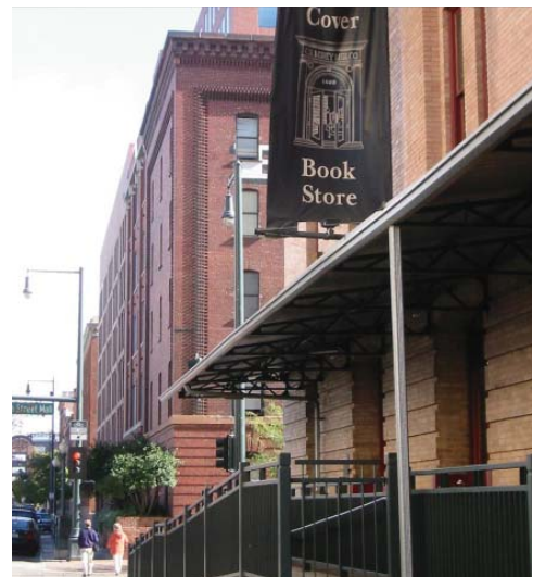
Figure 4-14: Example of an ADA ramp with shade structure.
