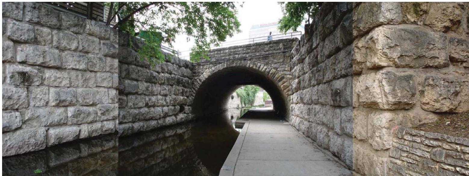
Approaching the 7th Street bridge
