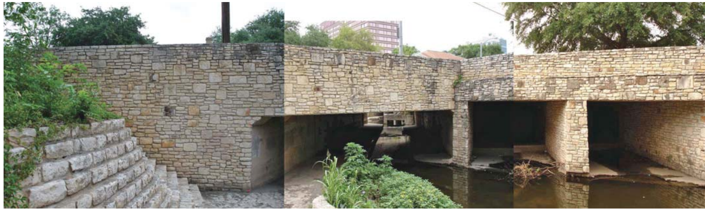
Looking east to Red River bridge
