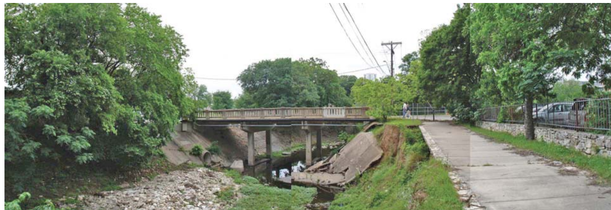
Looking south to 3rd Street bridge
