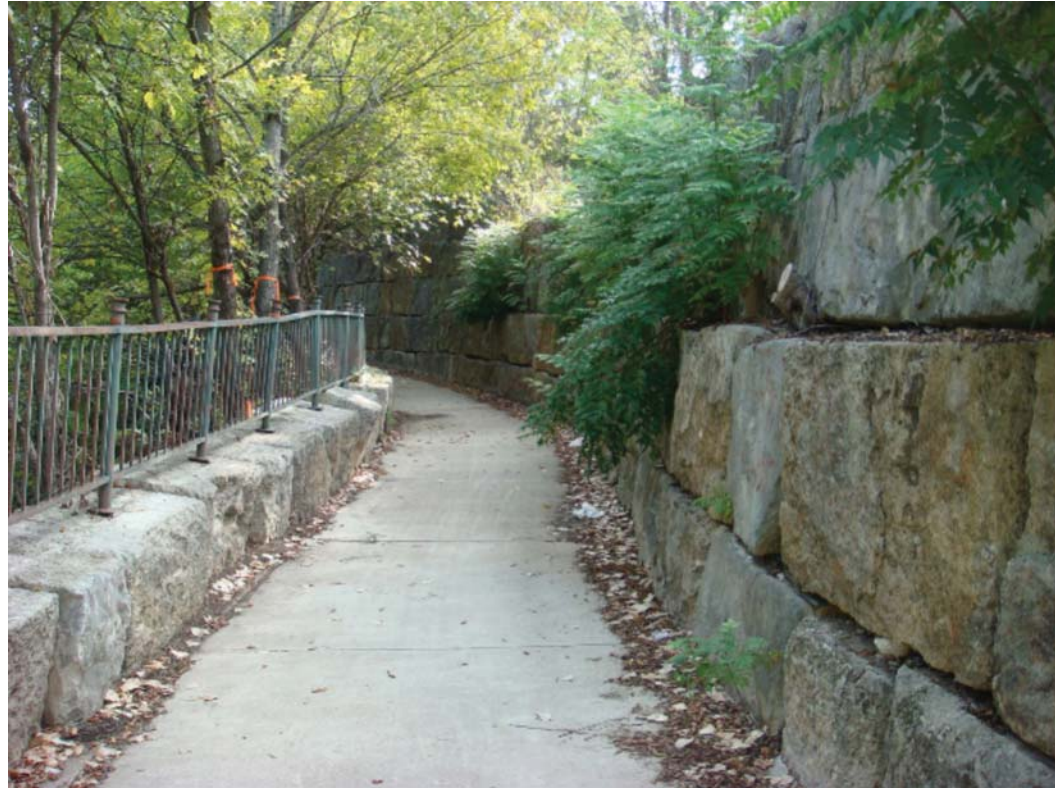
East bank of creek, south of Cesar Chavez
