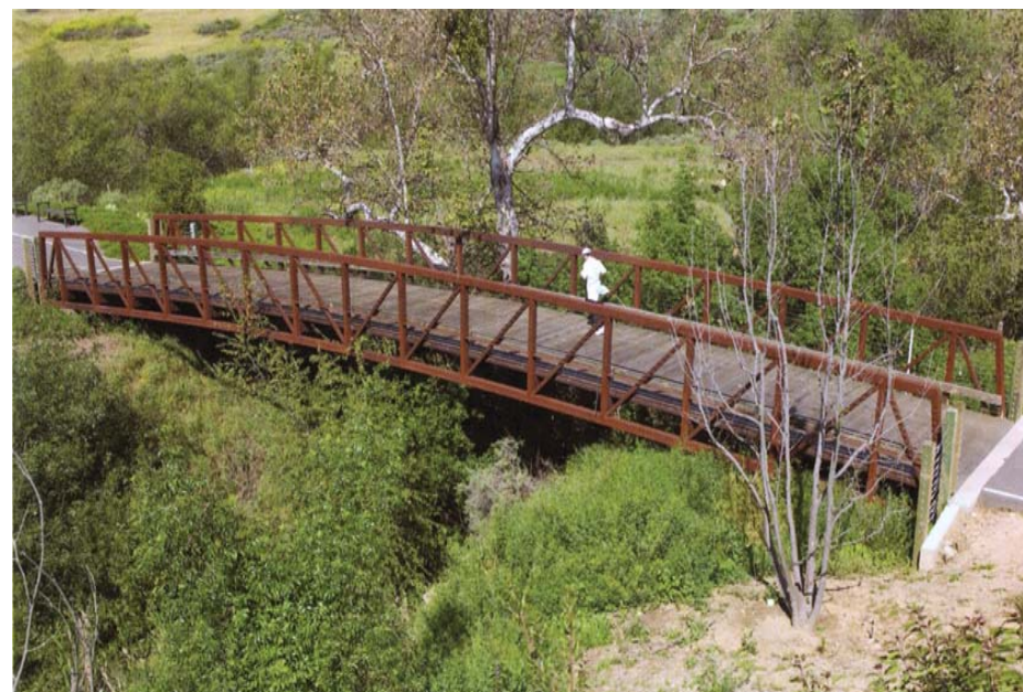
Sometimes a light bridge structure is required
