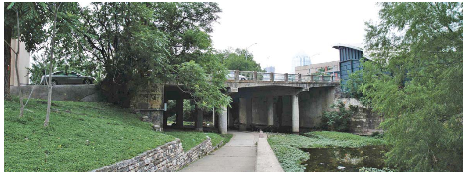
Looking south to 8th Street bridge
