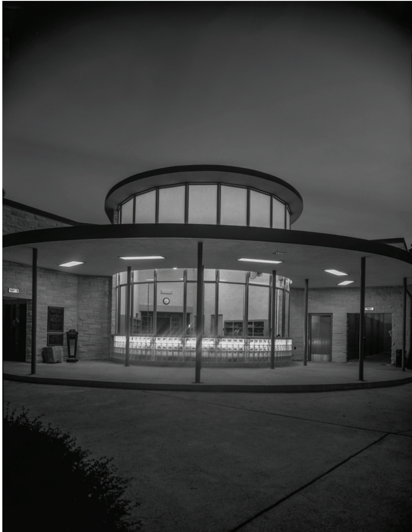
Barton Springs Bathhouse Rehabilitation
