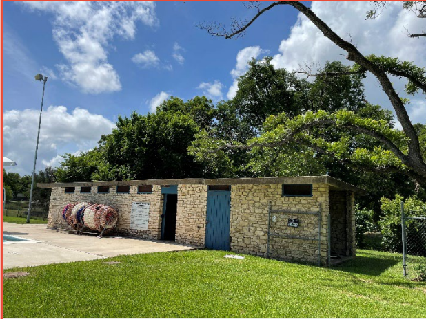
Mechanical and Storage Almacén
