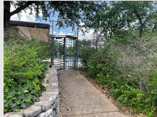
Exit Turnstile at North Torniquete de salida
