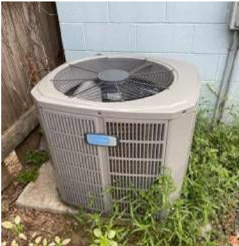
Equipment for the Quonset Hut
