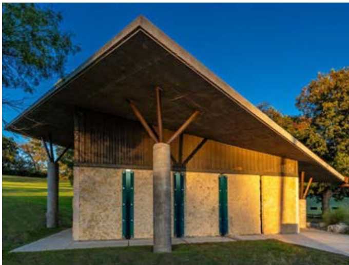
Zilker Park Trailhead Restrooms Source: 2021. Malla Photography
