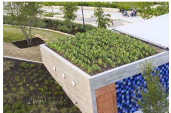
Example of Green Roof
