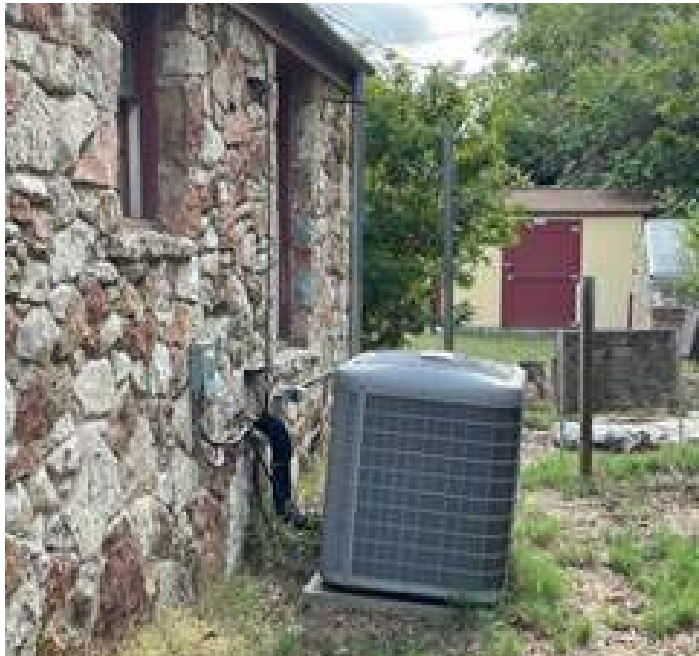
Ventilation of Caretaker's Cottage
