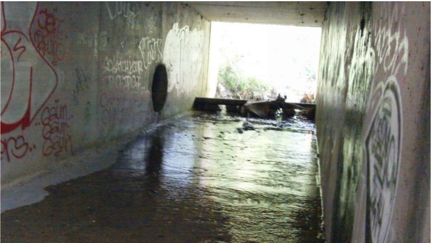
Location B.3a - Annie Street roadway culvert
