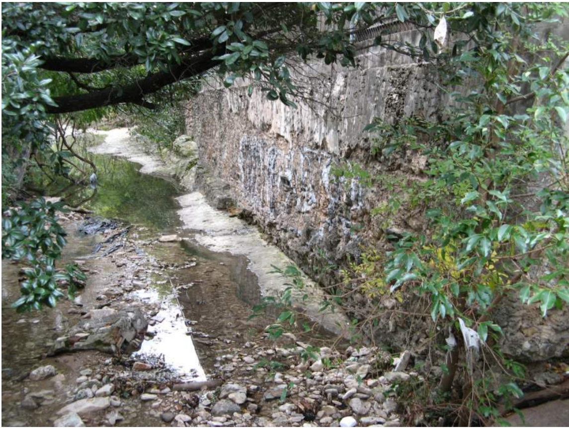
Location C.2 – East Bouldin Creek at Mary Street looking south
