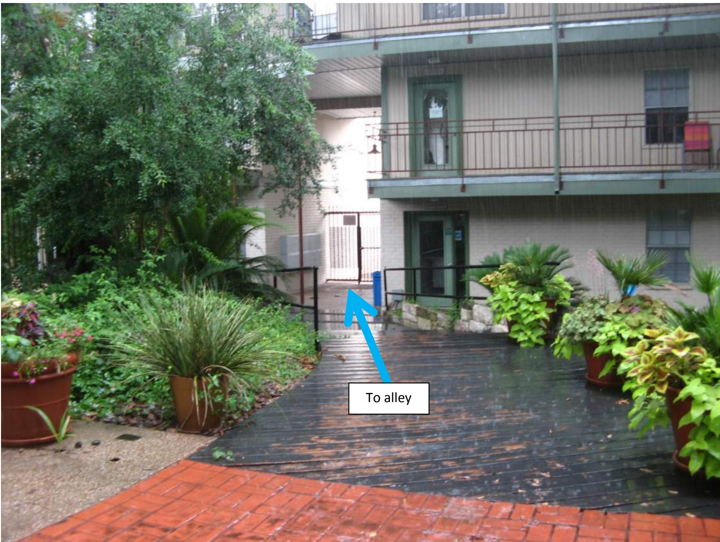
Interior courtyard drains under walkway to alley
