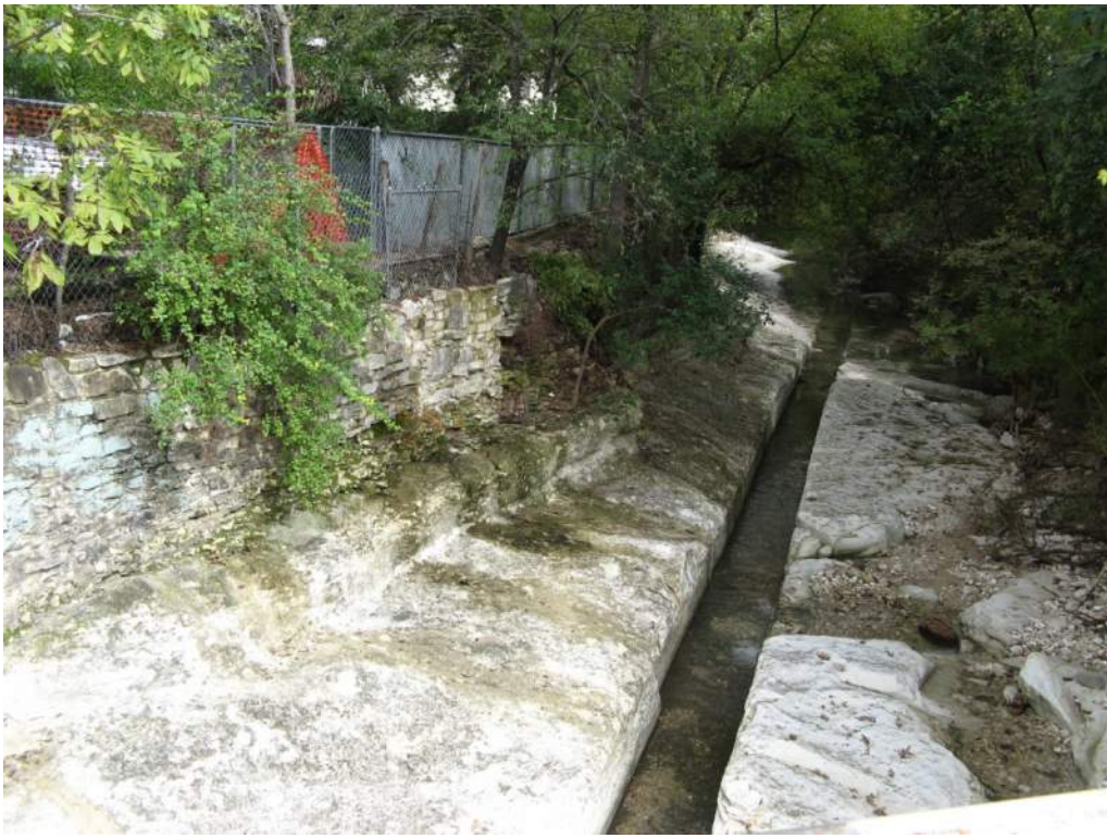
Location C.1 – East Bouldin Creek at Mary Street looking north
