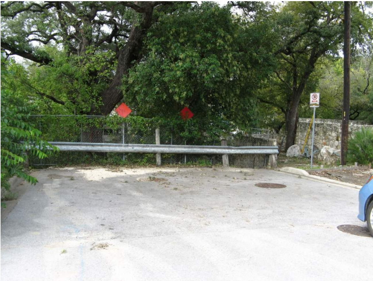
Location A.1 – Milton Street
