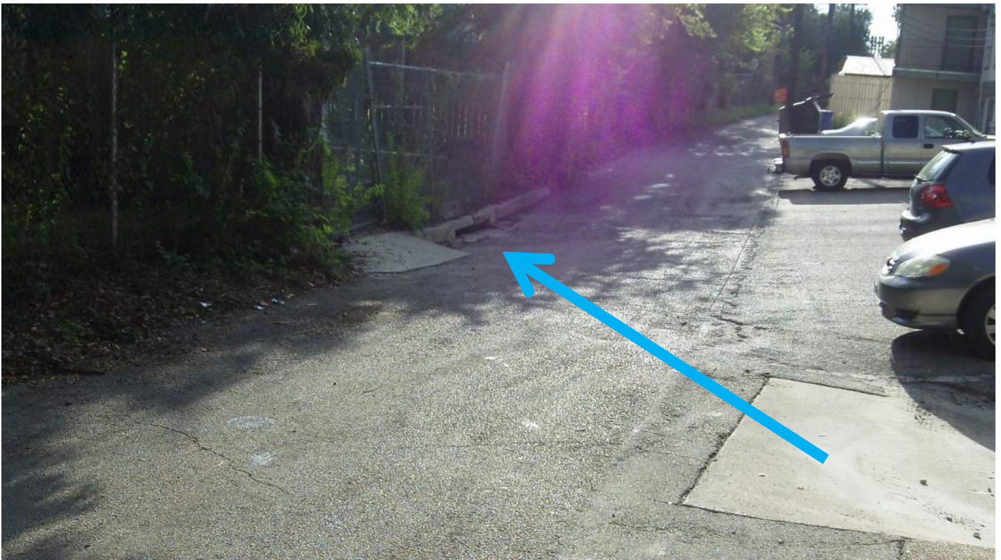
Courtyard runoff flows to sump inlet in alley
