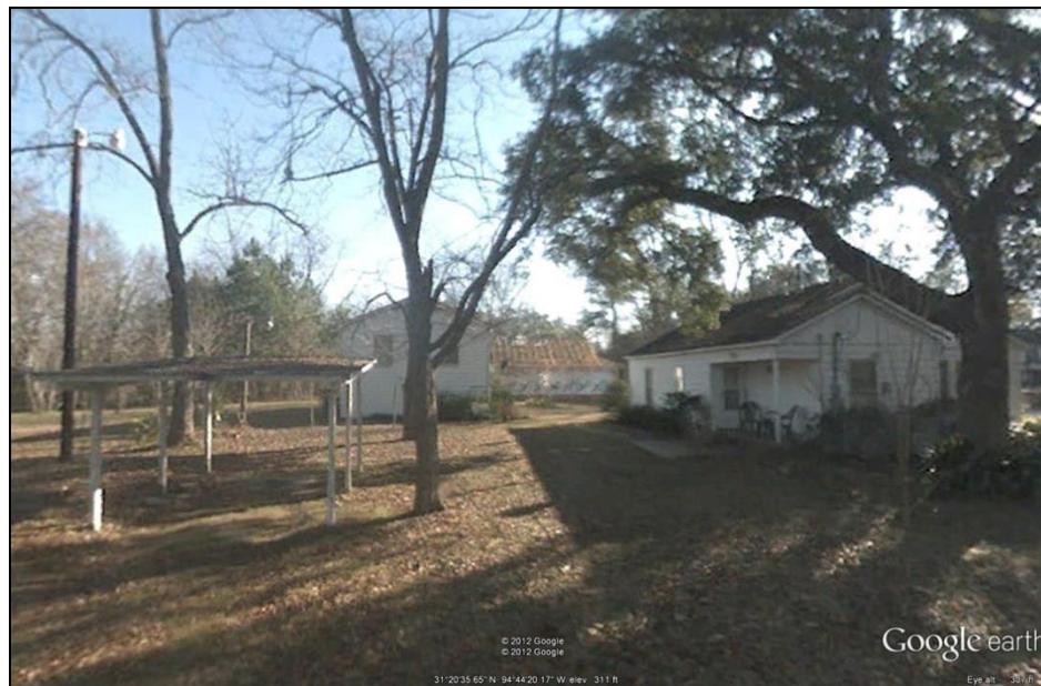
Side of home facing East (as seen from Google Earth street viewer).
